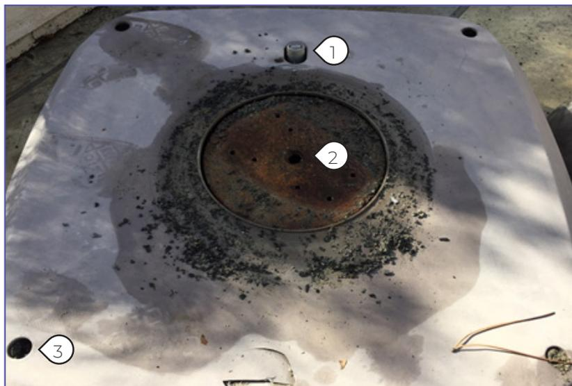
This is an OTU base which has rusted due to sea air (salinity) and a clear indication that it hasn't been maintained correctly.
